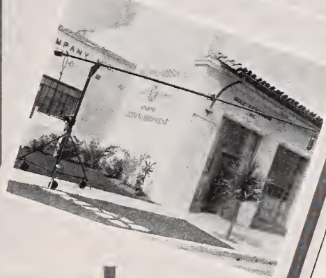
12. Mole-Richardson Bowl Lamp. This light was designed particularly to general large sets. The Bowl light is very popular with comedy producers, as they require a high intensity general illumination.
